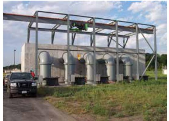
A worker shown in context with massive elbow bends at the discharge lines for the array of five, 100-mgd, 640-hp direct-drive Model PL7121 pumps supplied by Xylem's Flygt team. The massive units resolved effluent blockages once induced by high flows down the Missouri River.
