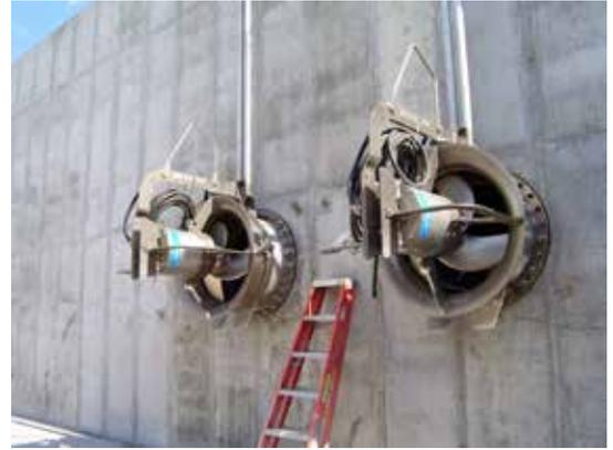
The retrofit changed the plant from an intrachannel design for secondary treatment to a design where two of the basins now rely on 40-hp Model SR4680 mixers that work in conjunction with a pair of Flygt PP4670, 20-hp recycle pumps that keep the anoxic zone mixed to desired ratios of homogenized influent, return activated sludge and recycled MLSS.
